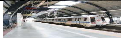
Common platform for all Metros
